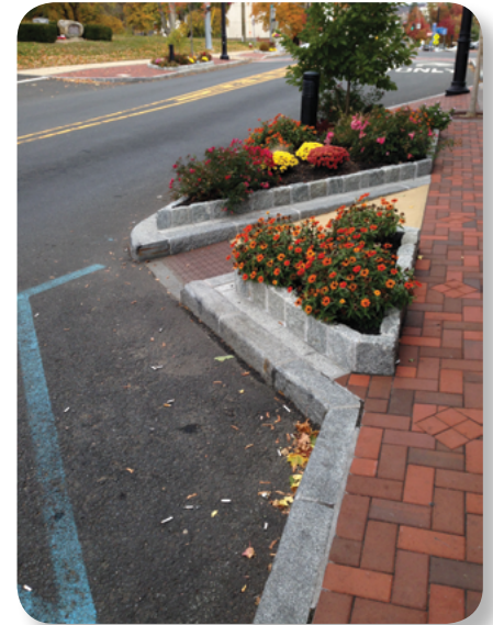
Access from the sidewalk to a parking space
