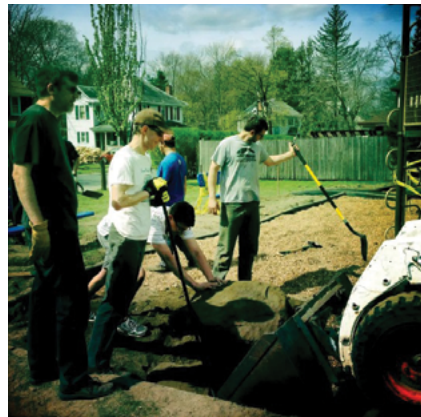
Beacon Playground Construction. Photo source: Caitlin von Schmidt
