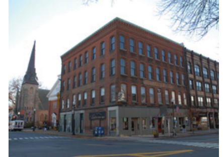
Arts Block in downtown Greenfield. Photo Source: VHB
