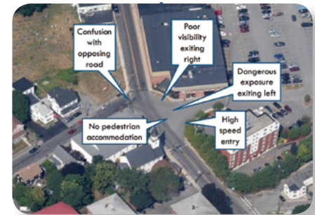
Woburn Downtown street improvement - Before
