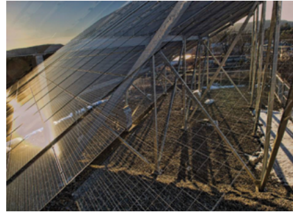
Solar panels on the John Olver Transit Center.
