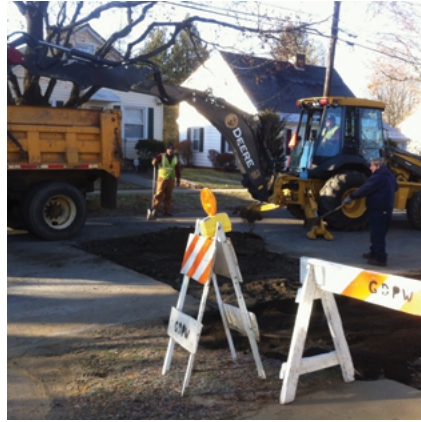
Greenfield DPW Staff hard at work. Photo source: Greenfield DPW.
