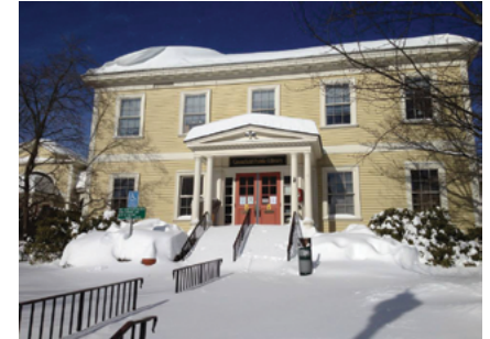
Greenfield Public Library. Photo source: Caitlin von Schmidt
