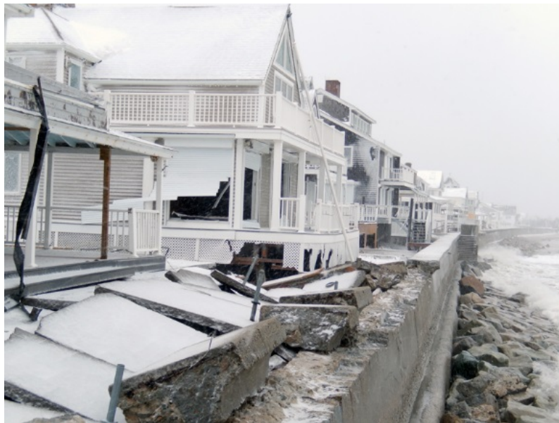
Photos of the seawall from the January 2015 Blizzard.
